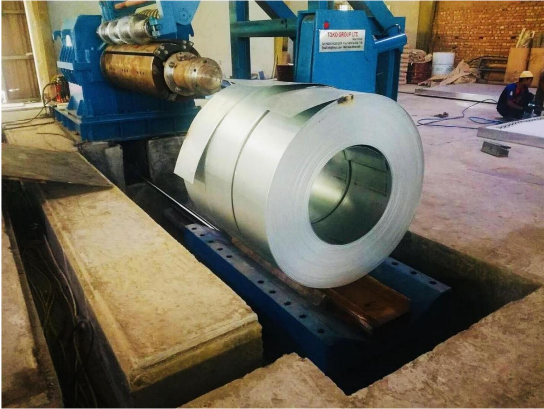
TOKO Slitting Line from Africa Customer's Factory
